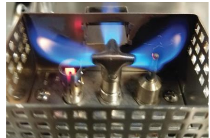
Figure 10.2 – Pilot flame coverage of thermocouple.
