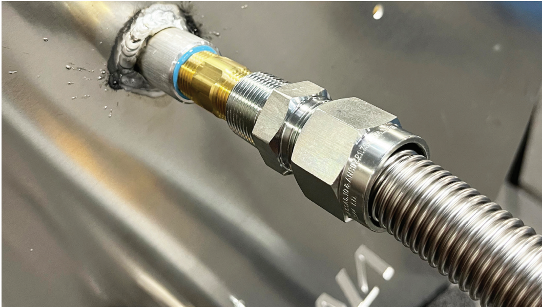
Photo 18: Connecting the Flex Line
