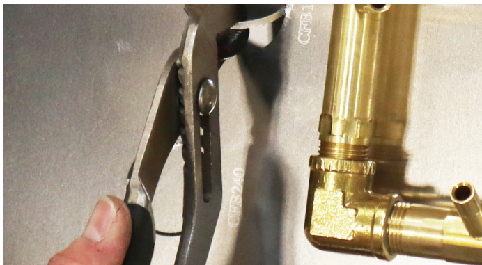
Photo 2: Breaking the Knockouts
